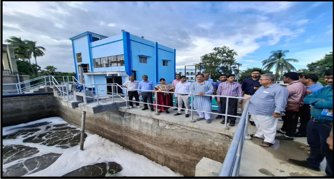
Photo of newly constructed STP at Sreenathpur, Ranaghat, Nadia
