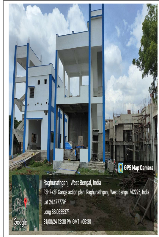
RAGHUNATHGUNJ STP SITE
