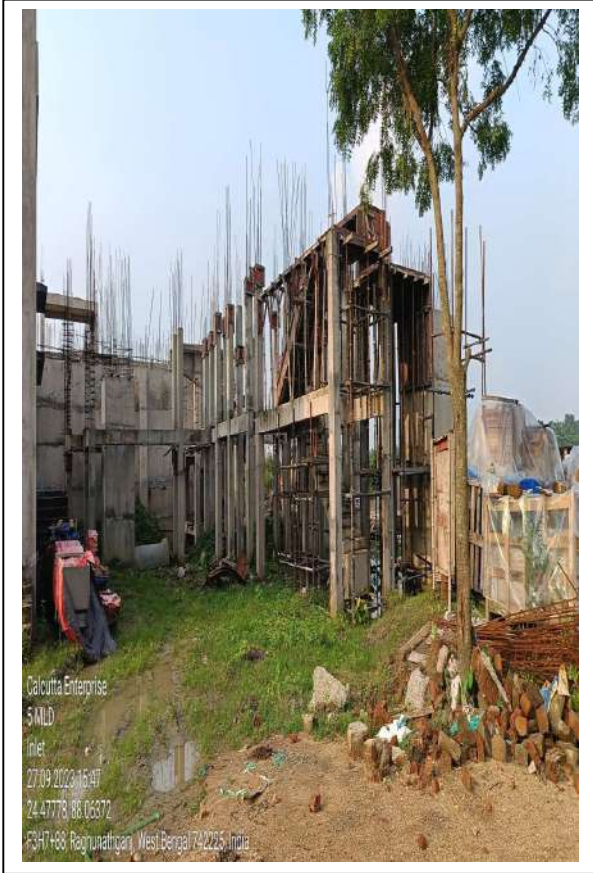
RAGHUNATHGUNJ STP SITE
